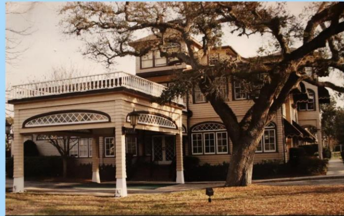
The Casements – northwest front view with extended canopy porch - ca. 2000.
