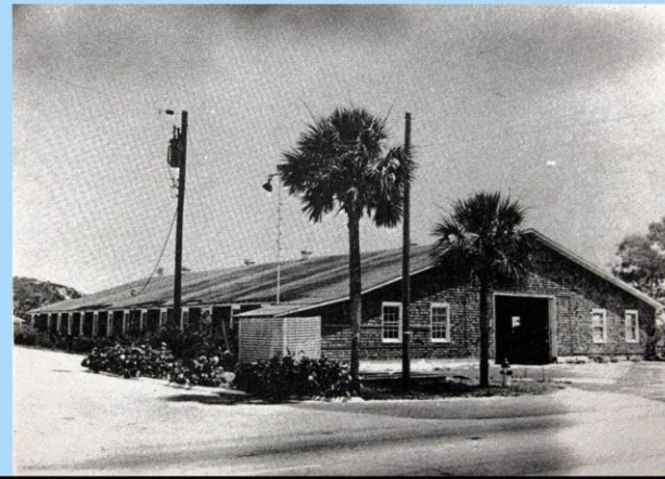
The Ormond Garage housed 100 automobiles. The historic structure burned to the ground in 1976.
